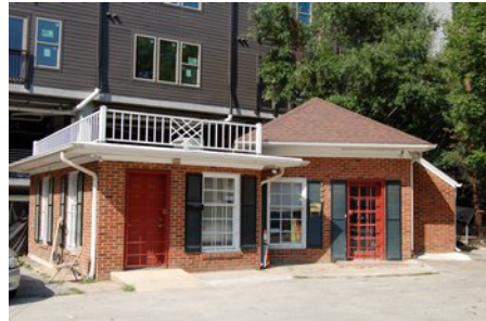
Building 2 – 1009 W Main
