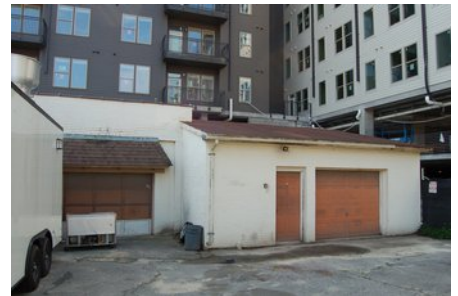
Building 3 – 1007 W Main
