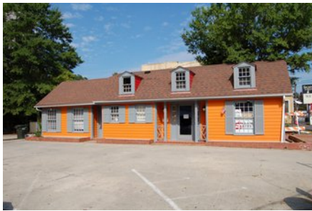
Building 1 – 1011 W Main
